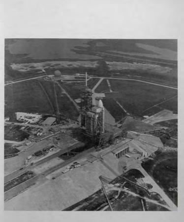
Figure 18. Rotating Service Structure in Access Position.
